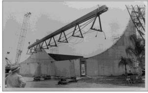
had yielded to Brutalism (from the French *beton brut*, or raw concrete). And instead of Glulam beams, the roof would be supported by cables hung from a 140-foot beam at the peak of the roof and anchored in the exterior buttresses on each side of the structure. The original plan called for the two main
